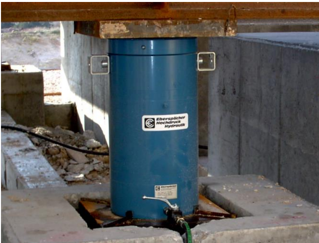
Hydraulic jack With adjustable locking ring
